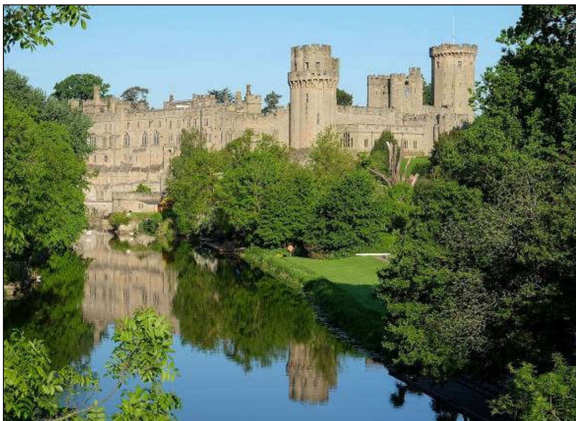
Greville was granted Warwick Castle by James I in 1604. The castle was in a dilapidated condition when he took possession and he spent £20,000 to restore it to former glory.
